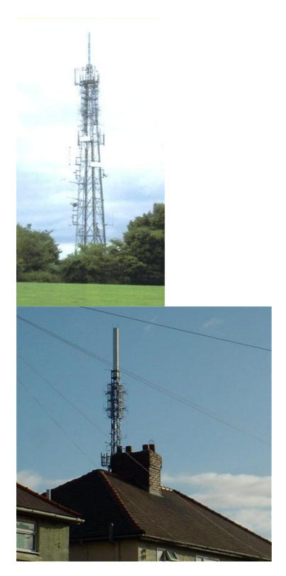
Each base station provides coverage over a limited area, or cell, in the area around the site. That's why in some countries mobile phones are called cell phones. To offer comprehensive network coverage, the cells must overlap each other like a patchwork quilt, so that users can move from one cell to another without breaking connection. As each cell can only handle a limited number of calls, the density of base stations has to be high in areas of heavy use.
